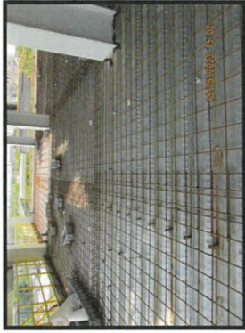
Installation wiremesh slab level +13.50 m. MP6.
