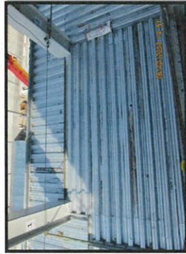
Installation the metal deck slab level +19.50 at MP7.
