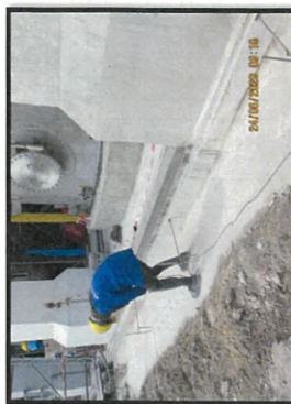
Breaking existing concrete slab for slab around MP6.
