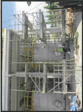
Pouring concrete pump foundation level +26.50 m. MP6.
