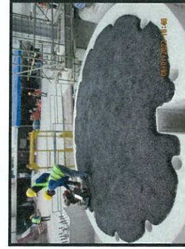
Installation the premixed asphalt of tank foundation no. T-9501.
