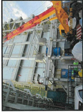
Installation the steel column line E/6 MP7 to level +19.50.
