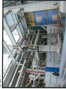
Installation the scaffolding for concrete encasing column
