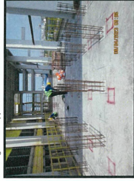
Installation column rebar with epoxy
