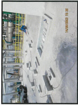
Pump foundation level +32.50 m. MP6.
