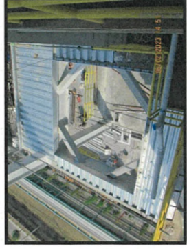
Installation the metal deck slab level +19.50 at MP7.
