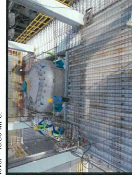
Installation the wiremesh for slab level +19.50 MP6.
