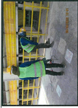
Installation column rebar with epoxy
