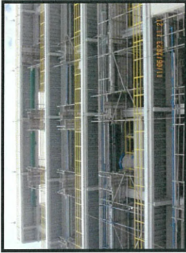
Installation pipe drainage level +19.50 m. +26.50 m. MP7.
