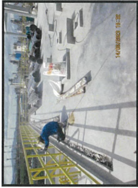
Remove gutter formwork level +32.50 m. MP6.
