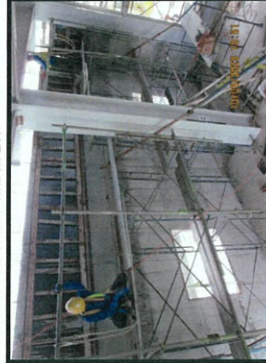
Installation the wall formworks of DCS room level +13.50 MP7.
