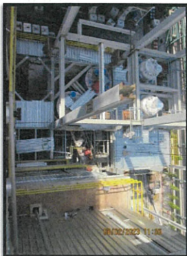
Installation the metal deck slab level +7.50 MP6.
