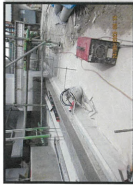
Breaking existing concrete slab for slab around MP6.
