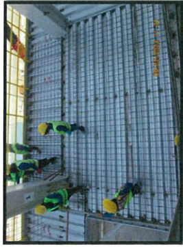
Installation wiremesh reinforcement level +19.50 at MP7.
