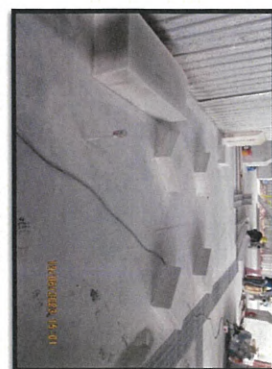
Pump foundation level +0.25 m. MP6.
