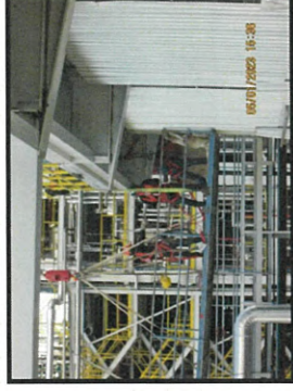
Installation the steel column line E/6 MP7 to level +19.50.
