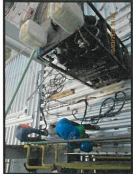
Welding the shear stud for metal deck slab level +26.50
