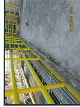
Installation the scaffolding for wall of MCC room and DCS room.
