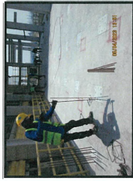
Installation column rebar with epoxy
