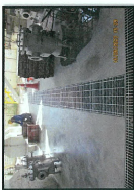
Installation galvanized steel grating +0.25 m. MP6.
