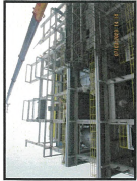
Installation the cantiliver beam frame level +32.50 MP7.
