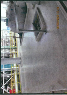
Liquid floor hardner level +19.50 m. MP6.
