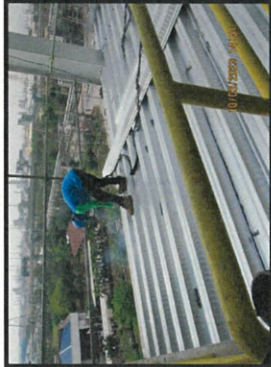
Welding the shear stud for metal deck slab level +26.50
