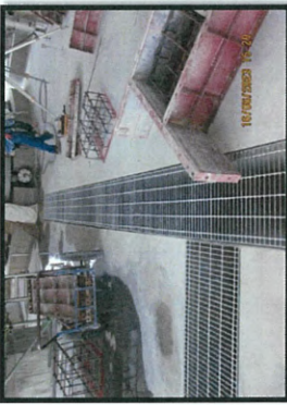
Installation galvanized steel grating +0.25 m. MP6.
