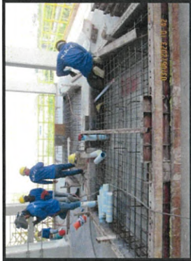
Installation rebar and formwork pump foundation level +26.50 m. MP6.
