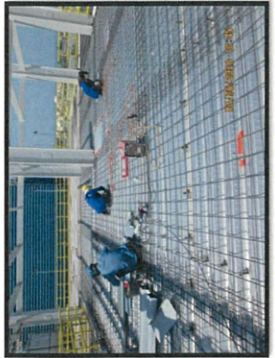
Installation gutter formwork level +32.50 m. MP6.
