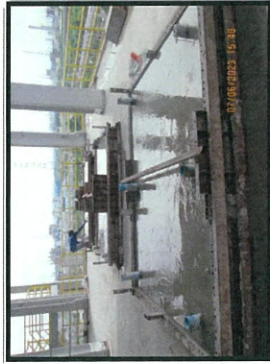
Pouring concrete pump foundation V-9558,V-9559 level +26.50 m. MP6.
