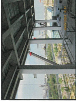
Installation the wiremesh slab level +38.375 MP7.
