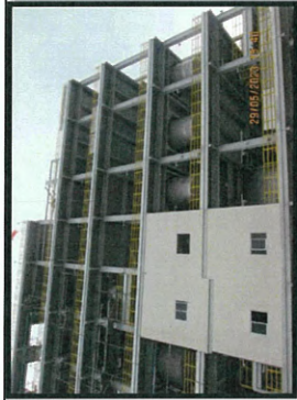
Installation aluminum glass window of DCS room and MCC room MP7.
