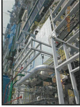
Installation pipe rack frame +35.608+36.80 m.MP6.
