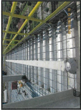
Installation gutter formwork level +32.50 m. MP6.
