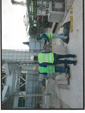
Installation the formwork for concrete encasing column at MP6.
