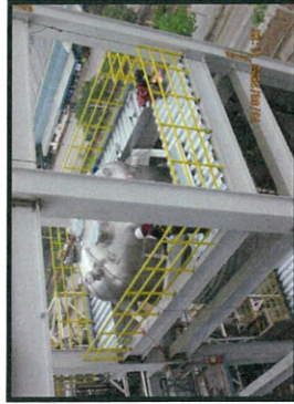
Installation the metal deck&handrail level +32.50 MP6.
