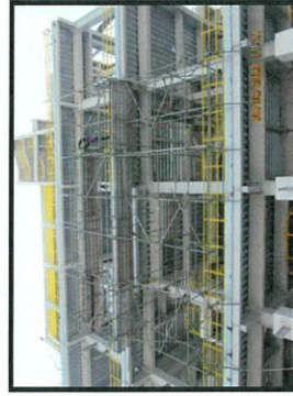
Installation the scaffolding for wall of MCC room and DCS room.
