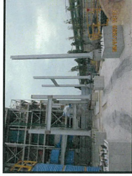
Installation the steel column MP6
