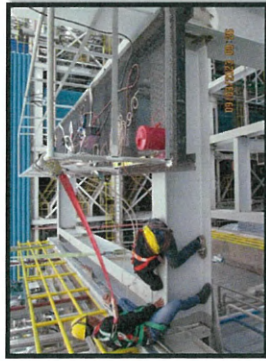
Installation the beam level +32.50 MP6.
