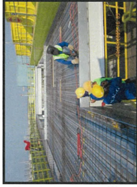
Installation the wiremesh slab level +38.375 MP7.
