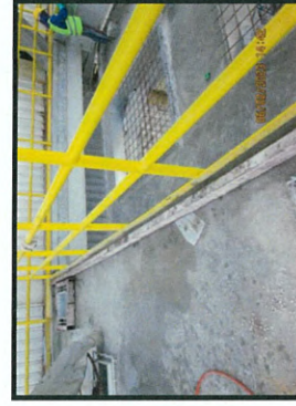
Pouring the concrete kerb level +13.50 MP7.
