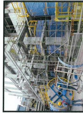
Installation the scaffolding for concrete encasing column
