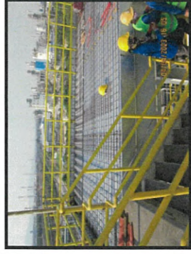
Installation the wiremesh slab level +38.375 MP7.
