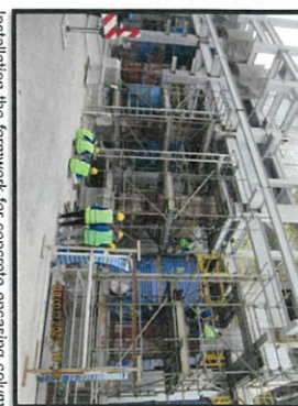
Installation the formwork for concrete encasing column at MP7.
