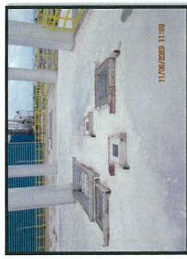
Installation grating tread of staircase to platform level +9.10 m. MP6.
