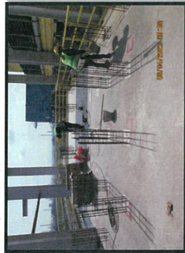
Installation column rebar with epoxy
