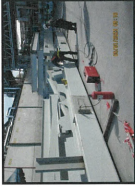
Installation the steel column line E/6 MP7 to level +19.50.
