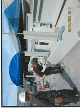
Welding the pipe rack at steel column.
