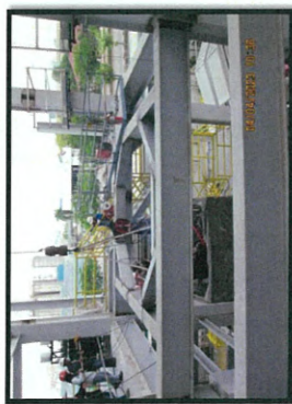
Installation the beam support for tank
