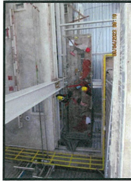
Installation the pipe rack level +24.80 +23.60
