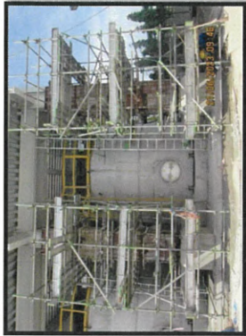
Pouring concrete column to 6 meters at level +0.25 m. MP6.
