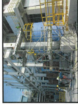
Installation the scaffolding for concrete encasing column at MP7.
