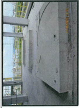
Remove formwork of pump foundation level +26.50 m. MP6.
