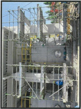
Remove column formwork and skim coating level +0.25 m. MP6.
