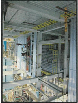
Installation the cantiliver beam frame level +32.50 MP7.
