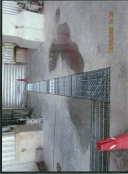
Installation galvanized steel grating +0.25 m. MP6.
