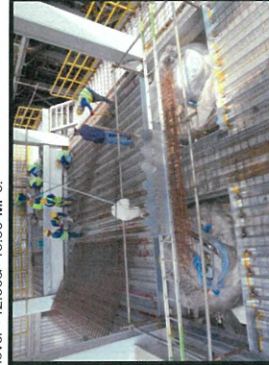
Installation the wiremesh for slab level +12.50&+13.50 MP6.
