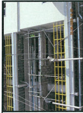
Installation PVC pipe rainage level +7.50 m. MP6.
