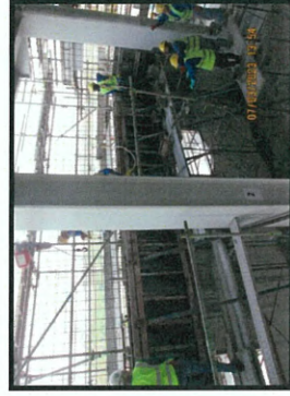
Pouring the concrete wall of DCS room level +13.50 MP7 on 7 March 23.
