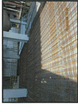
Installation wiremesh slab level +13.50 m. MP6.
