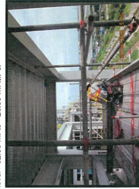
Welding pipe rainage support level +32.50 m. to +26.50 m. MP6.
