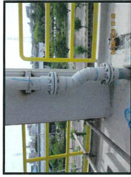
Installation pipe rainage level +13.50 m. MP6.
