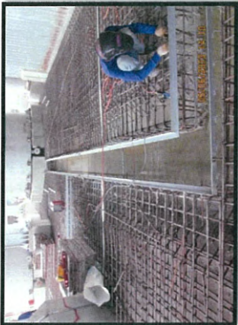
Installation angle bar of gutter level +0.25 m. MP6.
