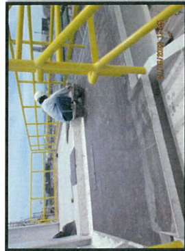
Installation granito floor tile level +32.50 m. MP6.
