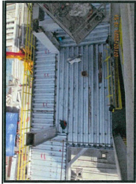
Welding shear stud at metal deck slab level +19.50 at MP7.
