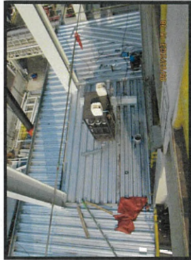
Installation the cantiliver beam frame level +32.50 MP7.
