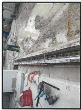
Remove column formwork and skim coating level +0.25 m. MP6.
