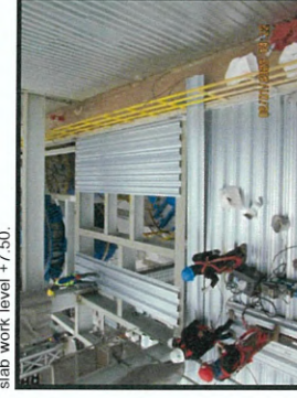
Installation the tempo.handrail for metal deck slab work level +7.50.
