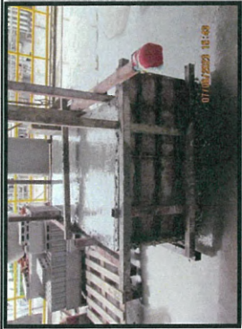
Pouring concrete pump foundation P-9561 level +7.50 m. MP6.
