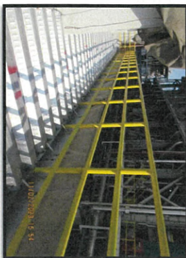
Installation the steel handrail and line marking for block out slab level +7.50 MP6.
