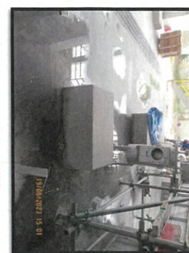
Pump foundation level +0.25 m. MP6.
