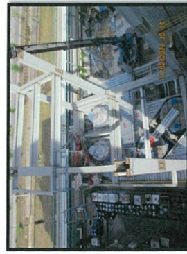
Installation the beam level +19.5 and metal deck slab level +7.50 MP6.
