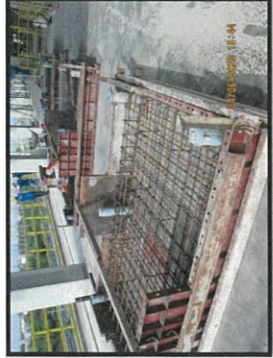
Installation rebar and formwork pump foundation level +26.50 m. MP6.
