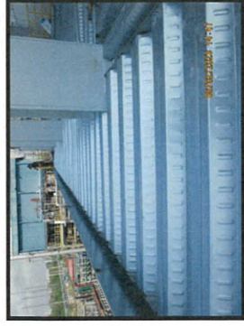
Installation the metal deck slab level +19.50 at MP7.
