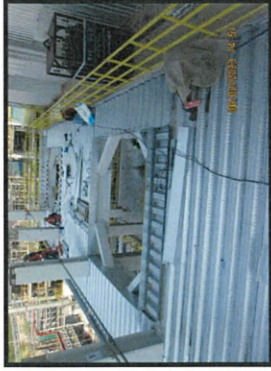
Installation the metal deck slab level +19.50 at MP7.
