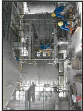
Installation scaffolding for column to 6 meters level +0.25 m. MP6.
