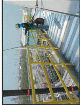
Welding the shear stud for metal deck slab level +26.50
